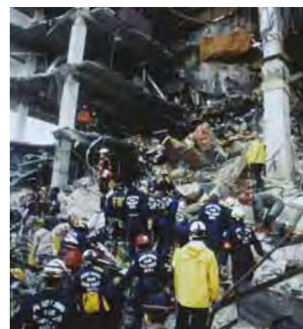
c. Structural collapse. The Oklahoma City bombing, 1995.
