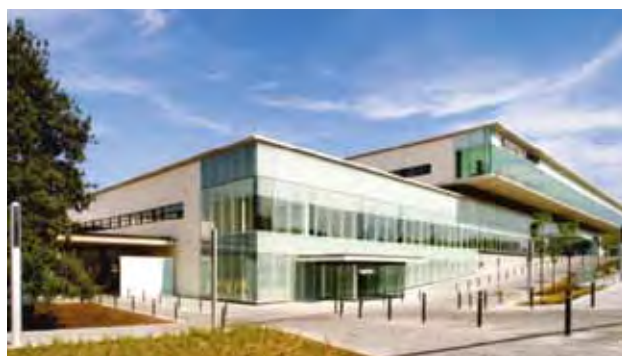
Hospital Le Mollet – Barcelona – Spain – bio-architecture and geothermic
