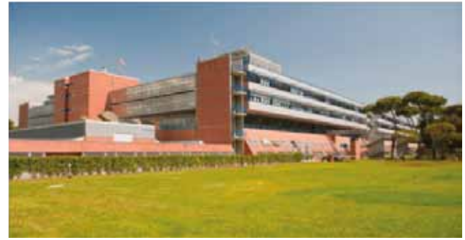
Hospital of Versilia (Lucca-Italy) - photovoltaic and efficiency
