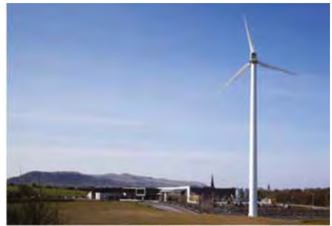
Girvan Community Hospital – Scotland (UK) – windmill and biomass-fuelled heating system
