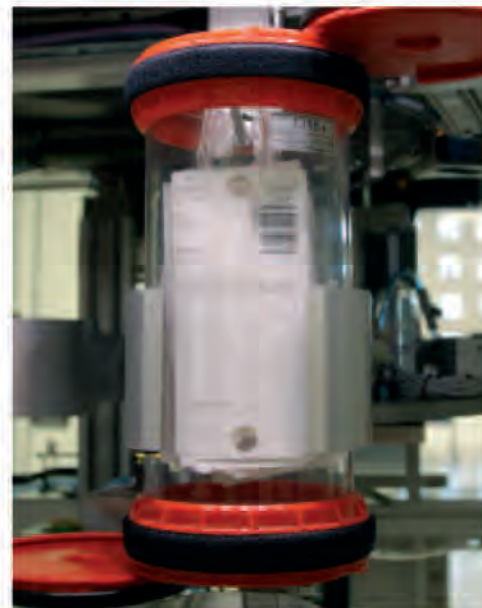
TranspoNet, the Pneumatic Tube System delivers therapy rings automatically to the wards
