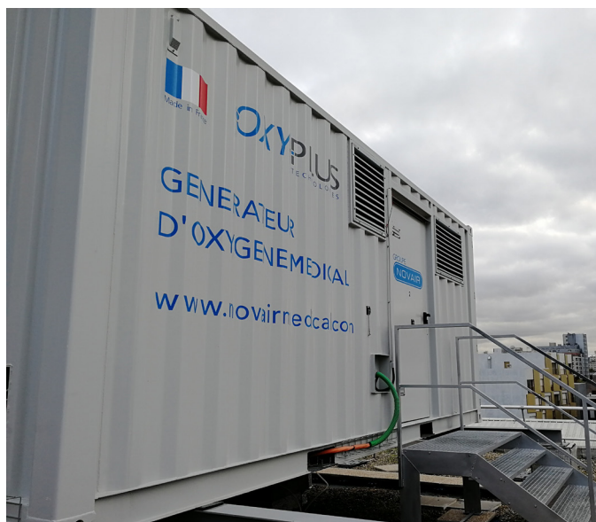
Caption : Containerized PSA oxygen plant installed on the roof of La Rosaie Hospital near Paris, France
